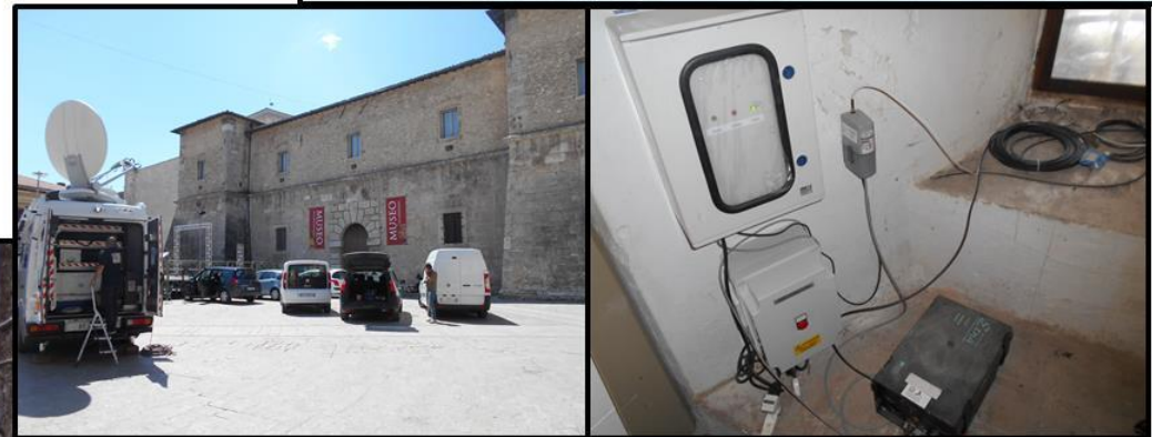
NOR - Norcia (at building's basement)
