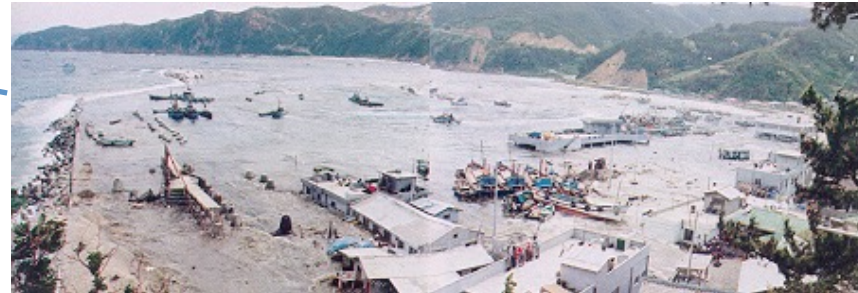
Damage of Tsunami(Imwon port)
