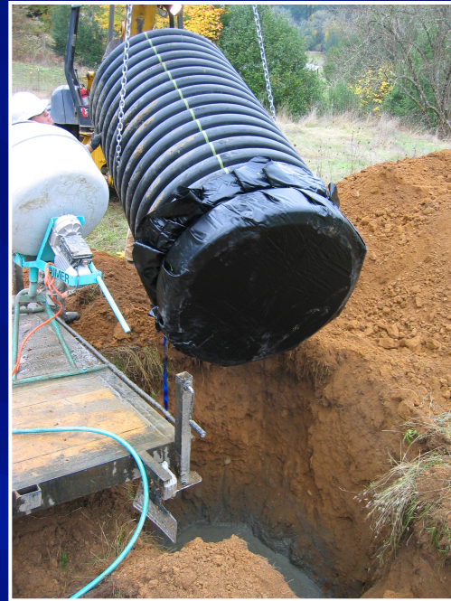
42" dia. pipe set into 7' deep pit with concrete on either side of rubber membrane
