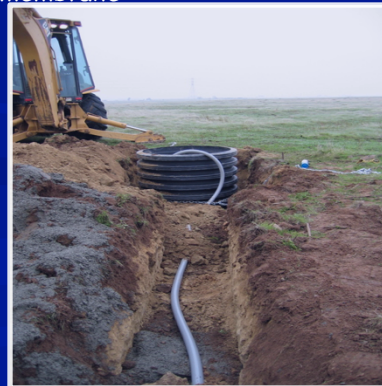
42" dia. pipe set into 7' deep pit with concrete on either side of rubber membrane
