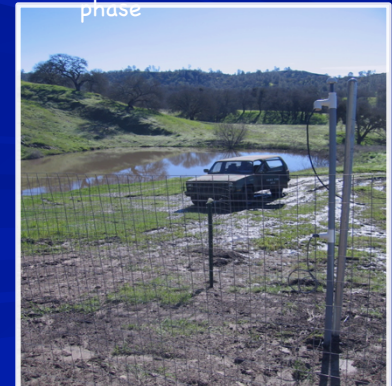
Flex conduit was replaced with straight sticks reducing field time significantly. Wires are pulled during construction phase
