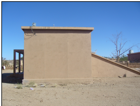
VBB Stations in operation
