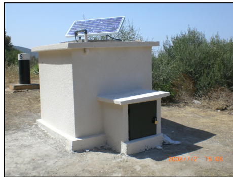
SP Stations in operation
