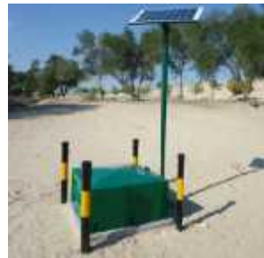
ADNOC Housing Ruwais
