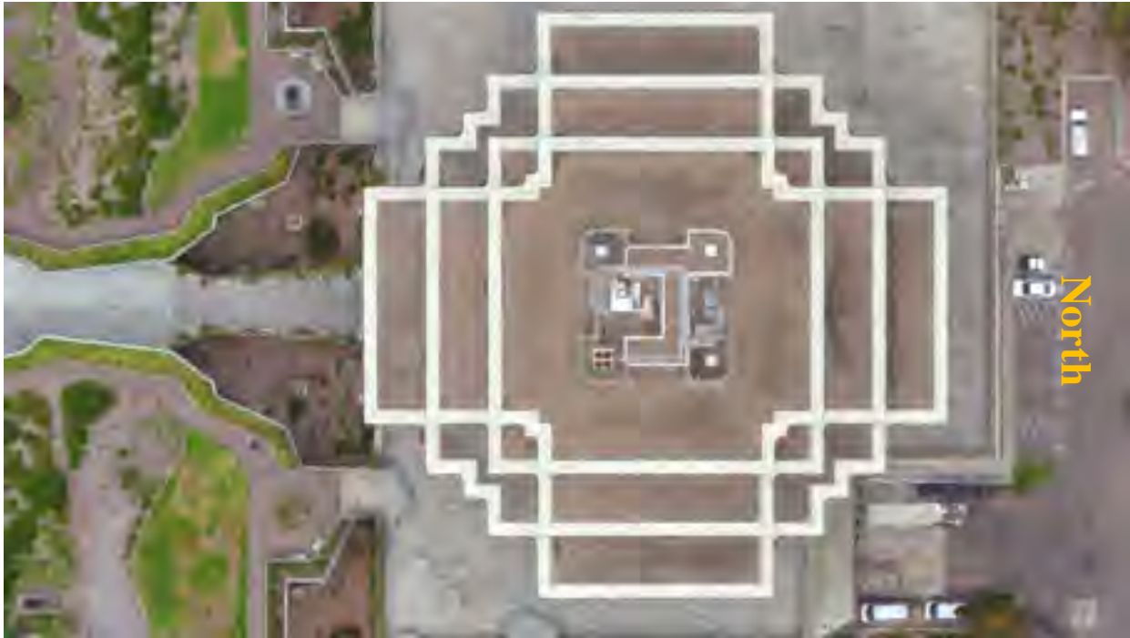
Top View of Library Rooftop
